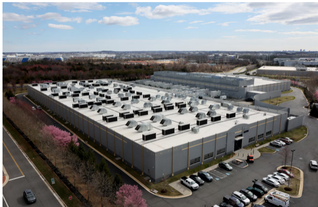
Figure: Digital Reality Data Center in Ashburn, Virginia, U.S.
